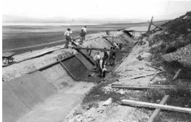
Photograph 11. Construction work on a concrete-lined portion of the Highline Canal Circa 1915.
