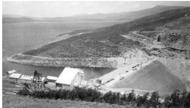
Photograph 8. Crushing and mixing plants from Reclamation Service's Salt River Project, Arizona, were erected at Strawberry during the Summer of 1911. Circa 1911.
