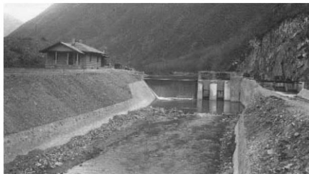
Photograph 6. Water was first diverted into the Power Canal on December 13, 1908. The gate keeper's house was added in 1909. Circa 1909.
