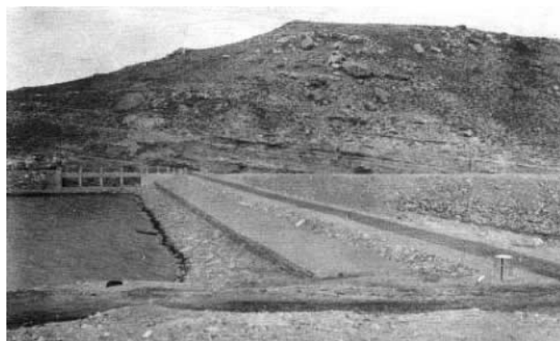
Photograph 9. Water starting to rise behind the newly completed Strawberry Dam. Circa 1915.
