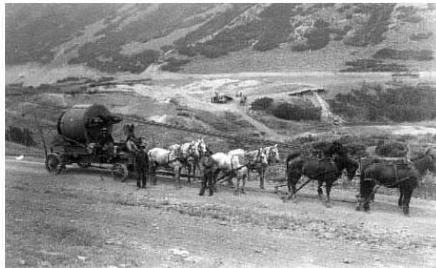
Photograph 4. The majority of the Power Canal traversed steep slopes and had to be concrete lined. Circa 1907.
