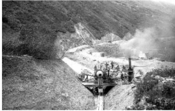
Photograph 3. The majority of the Power Canal traversed steep slopes and had to be concrete lined. Circa 1907.
