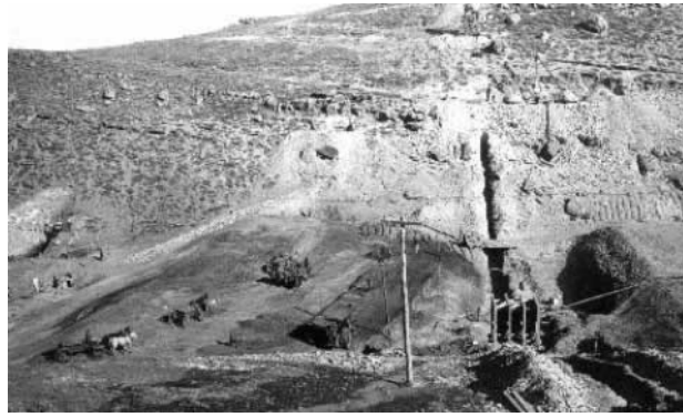
Photograph 7. While horse-drawn wagons delivered thousands of loads of earth fill to the Strawberry Damsite, the core wall trench was being excavated. Circa 1911.
